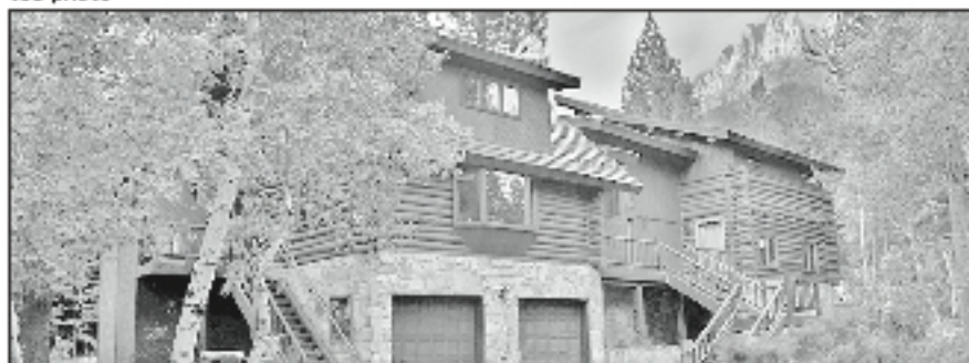
House in June Lake, front, retrofitted to incorporate geothermal heating. Submitted photo
